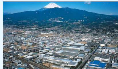
Meiden Numazu Works
