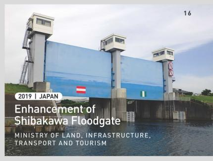
The Shibakawa Floodgate, which is a double-sluice gate type floodgate, was installed for the purpose of preventing floodwater from flowing back.
