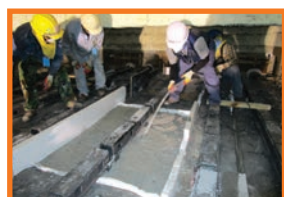
4. Lining (Refractory castable casting)
