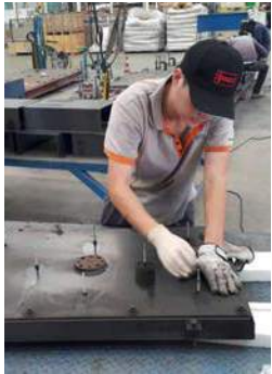
Repair of CFC Insulation
