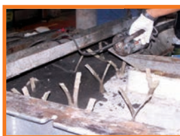
1. Install Support (Anchor)
