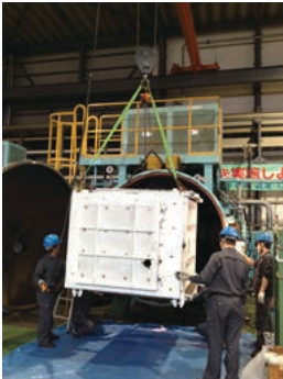
Overhaul of Hot Chamber
