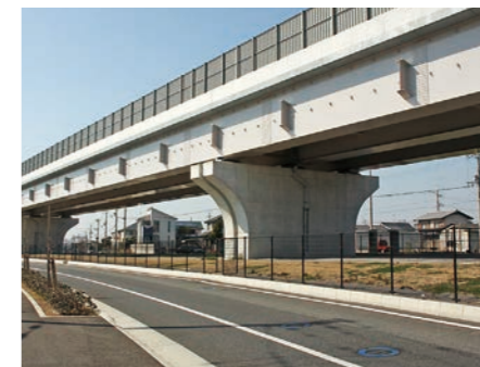
Higashiharima-Nanboku Road (Mizuashi Shintsuji No. 5 Elevated Bridge)
