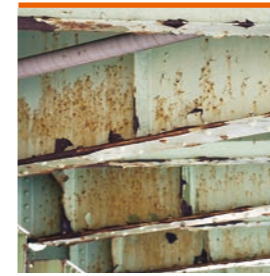
Peel-off of bridge coating (in an environment with severe salt injury)
