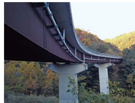
Ohama Grand Bridge (Oita Prefecture)
