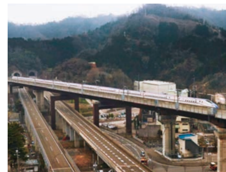
Hokuriku Shinkansen Hokurikudo Overbridge (Niigata Prefecture)
