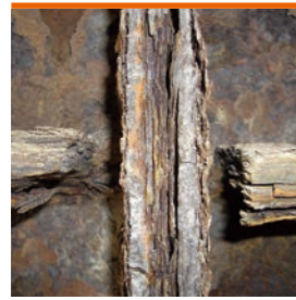
Corroding bridge (in an environment with severe salt injury)
