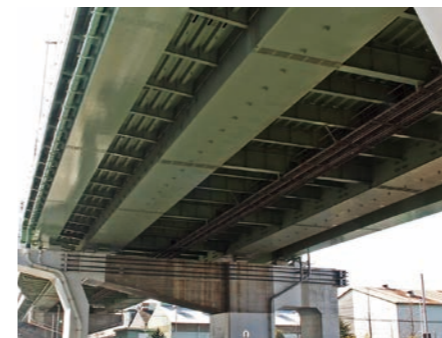
Hanshin Expressway Sambo Junction
