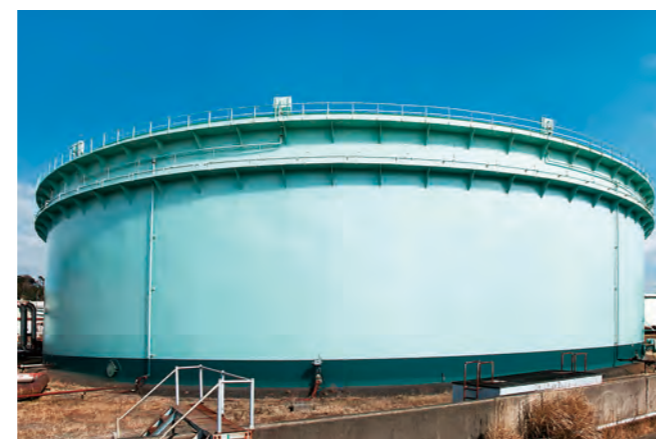
Crude oil storage tanks
