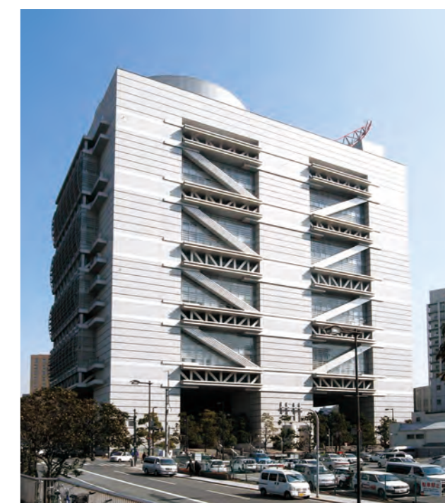
Conference center (application of steel Unbonded Braces)
